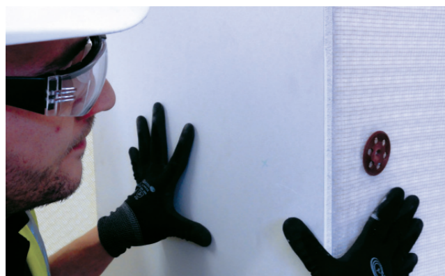
5 Apply wall finish
