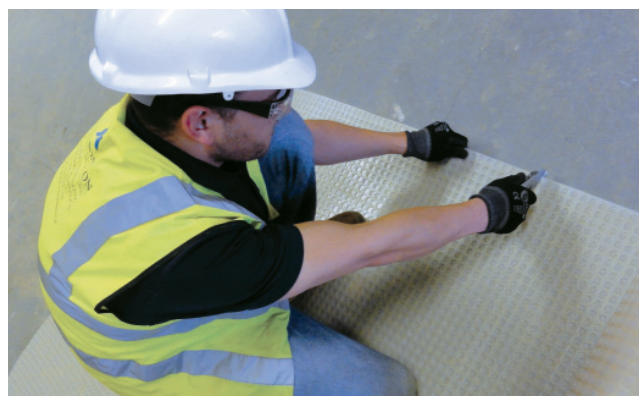
1 Cut the membrane to size
