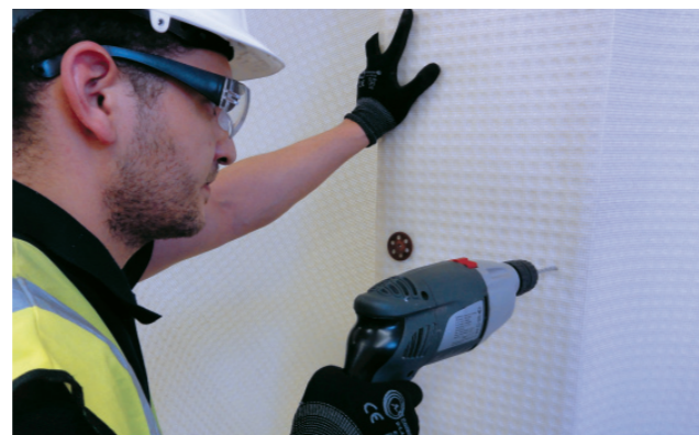
4 Drill and then fix with the fixing plug
