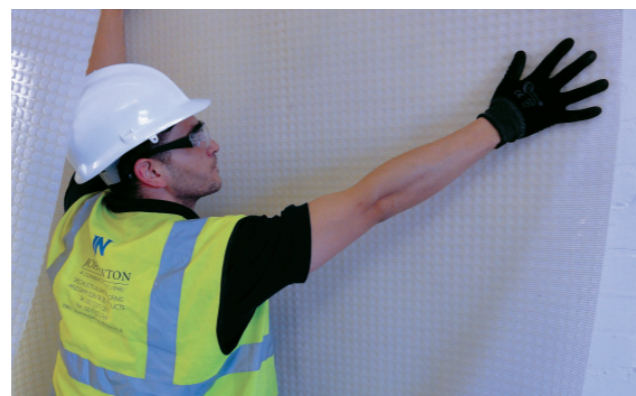
2 Place the membrane to the wall
