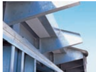
Laser-Line in use at Broad Green Hospital, Liverpool
