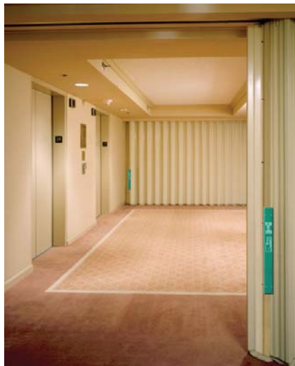
replace side-hinged doors for lift lobby protection/compartmentation...
