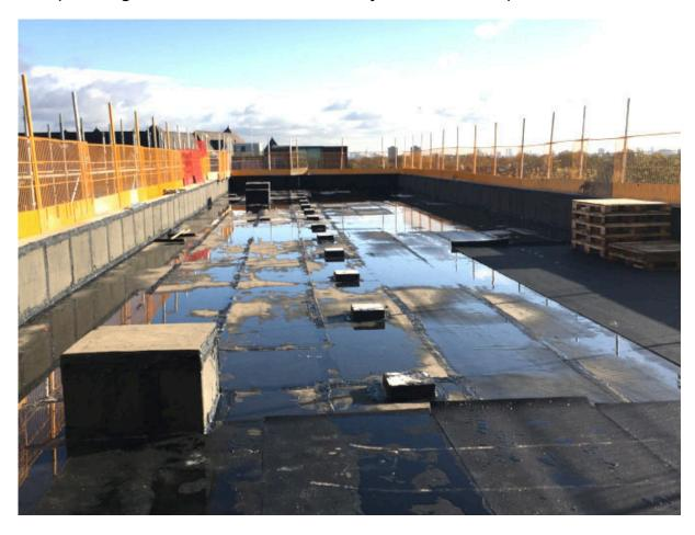
This membrane is completely rot-proof. It can be immersed in water without risk of delaminating or compromising its performance.
