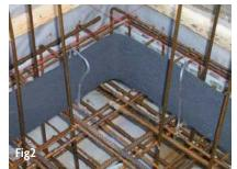
**CEMflex VB Plate** Waterstop may be installed by fixing it to the reinforcement using the **CEMflex Omega Holders** (as per figures 1 & 2) prior to pouring the concrete or alternatively **CEMflex VB Plate**
