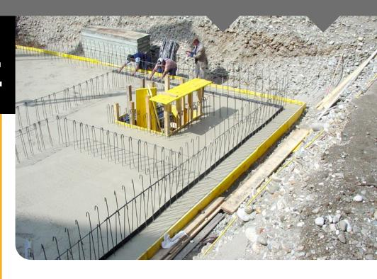
**CEMflex VB Plate Waterstop** consists of a galvanized steel plate encapsulated in a special patented coating which reacts with water to provide a watertight joint, for use in all non-movement construction joints in reinforced concrete. CEMflex VB complies to BS 8102:2022
