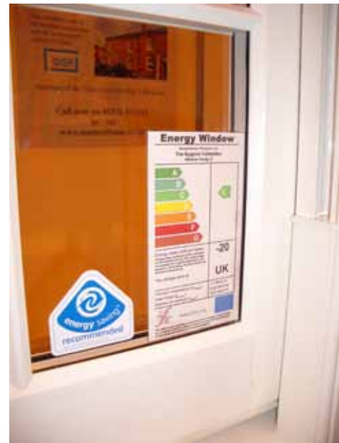
Figure 7.3 Windows are rated on an A to G scale. Picture: BRE.
