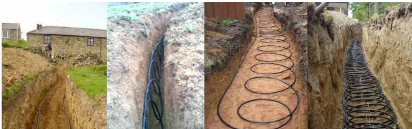
Figure 10.3 Ground loops for ground source heat pumps
