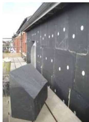
Figure 6.4 The 250 mm thick external wall insulation, with a block shaped to fit at the eaves. Picture: Simmonds Mills Architects.
