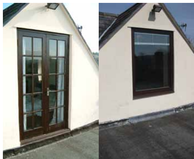
Figure 3.2 Door replaced by a window to accommodate future flat roof insulation. Pictures: John Willoughby.
