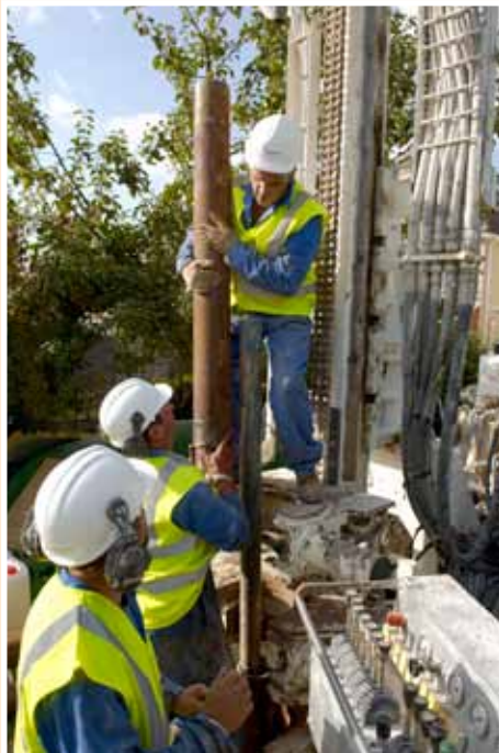
Installing the ground source heat pump
