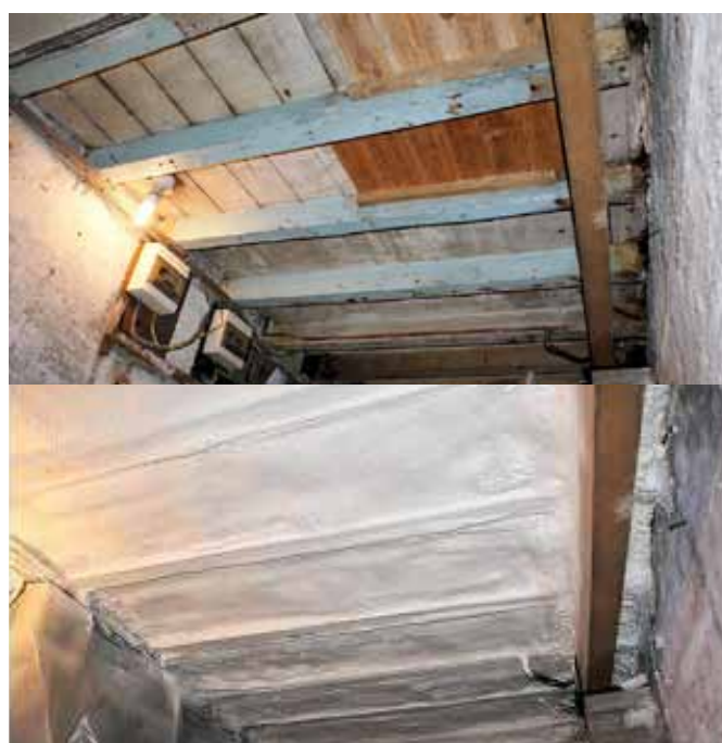
Figure 4.5 The floor seen from the cellar; before and after the installation of spray-applied polyurethane insulation. Pictures: Isothane.
