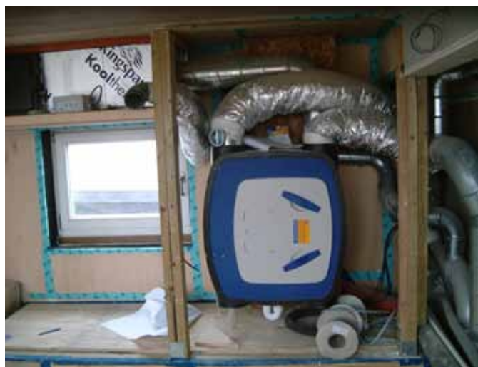
Figure 9.7 Heat recovery ventilation in a refurbishment project in Hackney (note the conglomeration of ducts and also the extensive use of sealing tape). Picture: John Willoughby.
