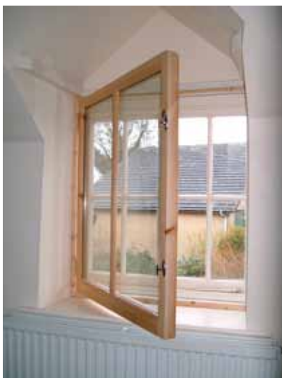
Figure 7.6 Using 4/6/4 mm low emissivity krypton filled glazing gives a high performance for this handmade secondary window. The overall U value is about 1.2 W/m²K. Picture: John Willoughby.
