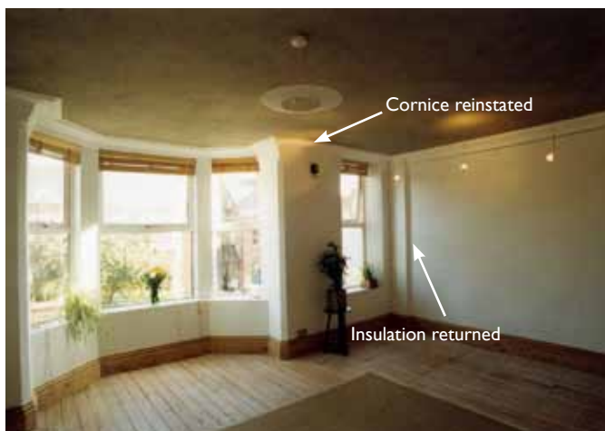
Figure 5.17 Internal insulation at the Nottingham EcoHome – note the reinstated coving and the insulation returned along the party wall. Picture: Gil Schalom.
