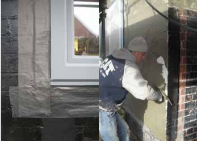
Figure 8.7 Windows taped to walls before they were rendered and covered with 250 of insulation. Pictures: Simmonds Mills Architects.
