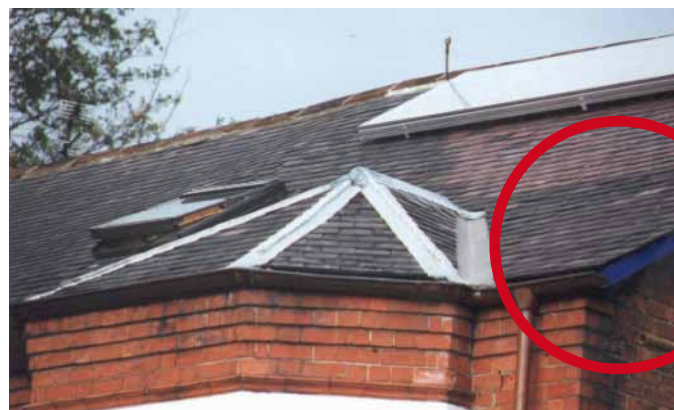
Figure 3.1 Extended roof verge to accommodate future external wall insulation. Picture courtesy of Gil Schalom.
