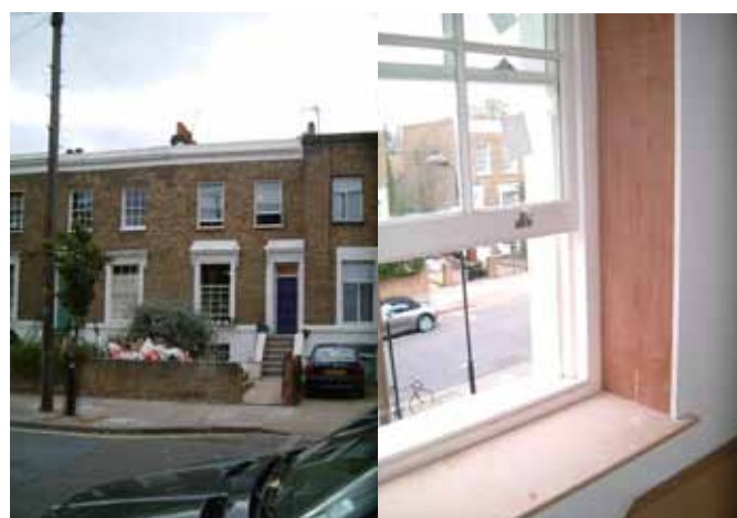
Figure 8.5 Exceptional levels of air-tightness have been achieved at this refurbishment project in Hackney. New draught-proof windows have been carefully sealed to new internal wall insulation. Pictures: John Willoughby.
