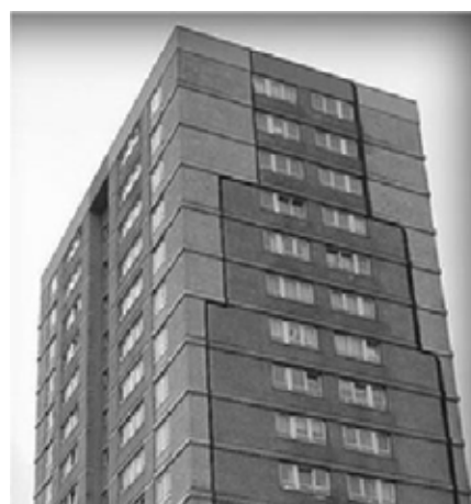
Figure 5.3 A high-rise block in Edinburgh insulated with proprietary polyurethane cavity wall insulation. Picture: Isothane.
