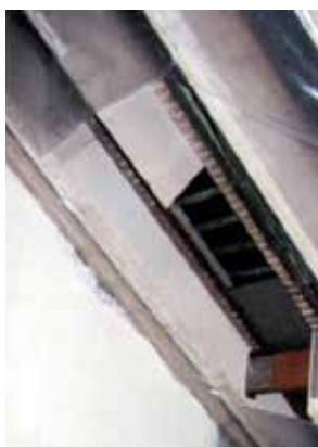
Figure 6.8 Recess for rooflight in 300 mm deep extension rafters with air/vapour barrier and plasterboard. Picture: Gil Schalom.
