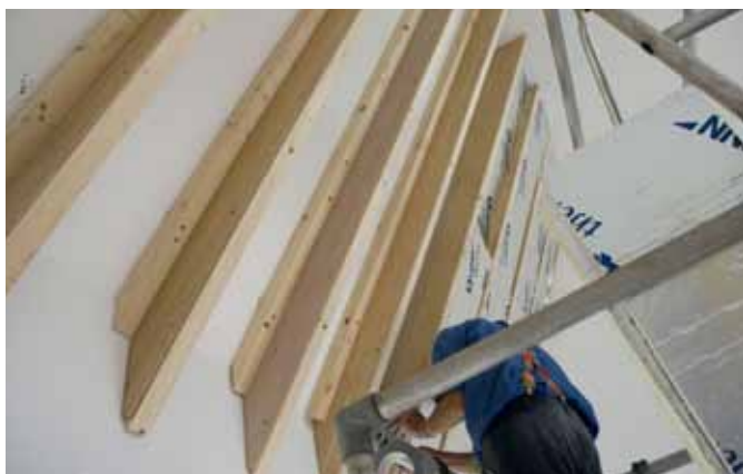
Figure 6.6 Z rafters were set out using a jig to ensure the spacings matched the rigid insulation board. Picture: Ray Exton.
