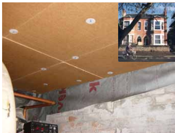
Figure 4.3 Insulating a suspended floor from beneath, at the Nottingham Ecohome. Picture courtesy of Gil Schalom.
