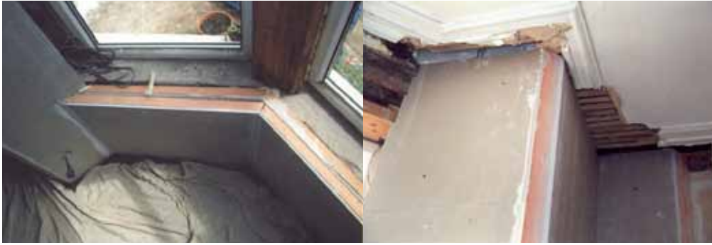
Figure 5.15 Internal insulation at the Nottingham EcoHome. Pictures: Gil Schalom.
