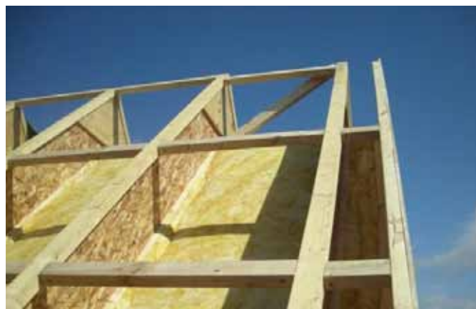
Figure 6.3 400 mm deep engineered timber 'I beams' with the first layer of roof insulation over the existing roof structure. Picture: Simmonds Mills Architects.
