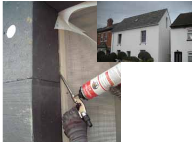
Figure 5.8 The gap between 250 mm thick grey polystyrene insulation and a window frame being sealed with expanding foam prior to rendering at Grove Cottage, Hereford. Pictures: Simmonds Mills Architects.
