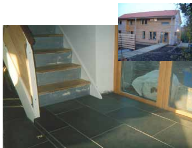
Figure 4.9 A landing built at the bottom of stairs to even out the risers. Pictures: Tony Cleford.
