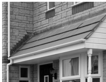
Type G provides the horizontal protection and Type X the stepped protection
