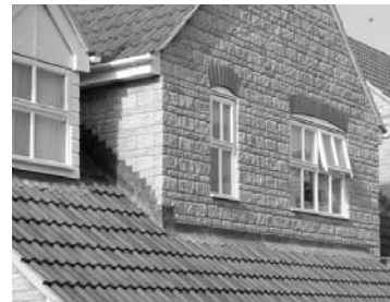
Type G cavitytrays with attached lead flashings provide protection to the front horizontal intersection. Note the Type X trays used above the sloping abutment terminate with an external angle. This provides a protective link with the Type G trays.
