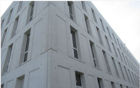
Cast-in-place concrete construction
