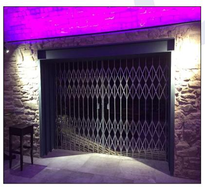
Spearhead gates run on a flat bar bottom track which is folding or portable. The top track is a folding or portable flat bar. The weight of the gate is supported by pulleys at the base of the pickets.
