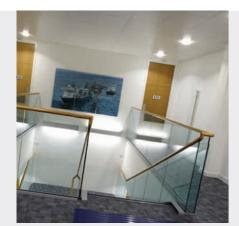
This commercial installation featured Crystal with Natura handrails on the stairs, Jasper with Natura handrails in the restaurant area and Crystal with Onyx handrails in the exterior bridge area. We also manufactured the bridge itself.
