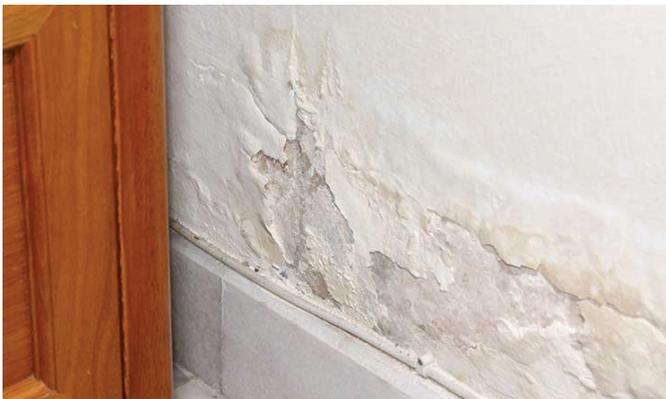
Dampness as a result of hygroscopic salts without any free or capillary moisture, is often referred to as salt damp. Visual evidence of salt damp will be dependent on humidity levels. Hygroscopic salt contamination of the plaster work may sometimes be detected with the aid of an electronic moisture meter even if the surface appears visually dry.
