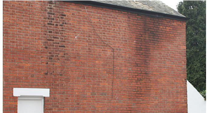
A full understanding of the distribution of dampness in a structure will normally require the use of various moisture measuring techniques. Surveyors should be familiar with the use of such equipment and interpretation of the results produced. It must be recognised that electrical moisture meters will produce only qualitative and comparative readings in masonry. These readings may also be affected by salts.
