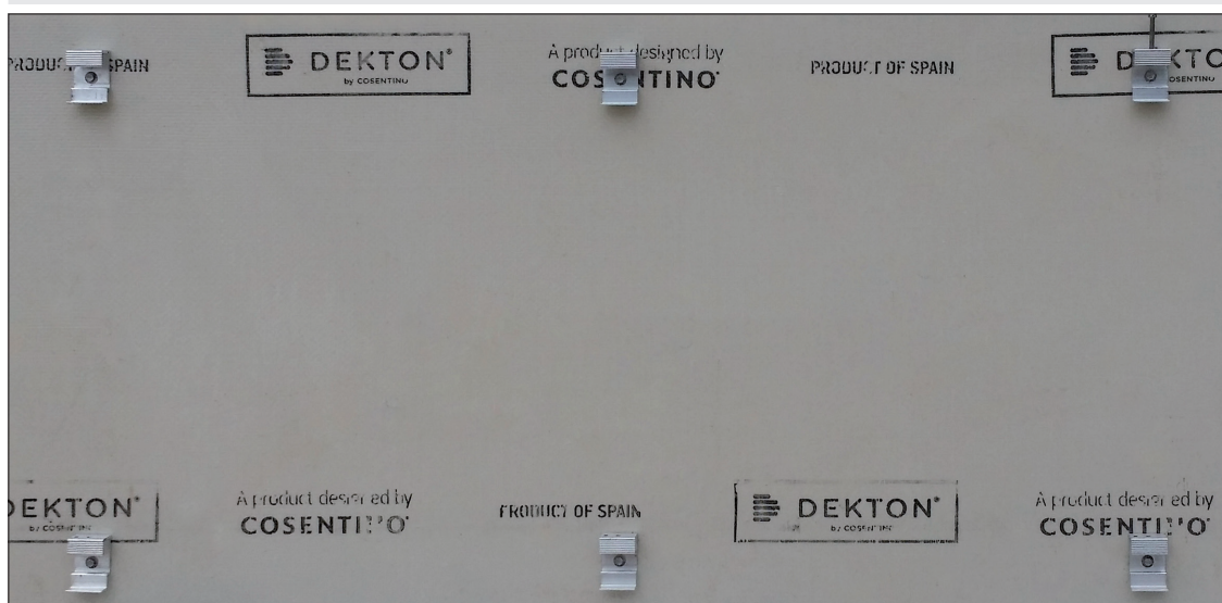
Figure 2 Panels with Keil Anchors fixed into undercut drill holes
