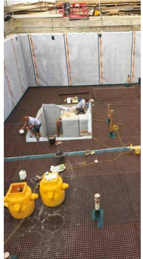
One of the main design considerations when designing a Cavity Drain System is to consider managing the collection and discharge of ground and/or foul water.
