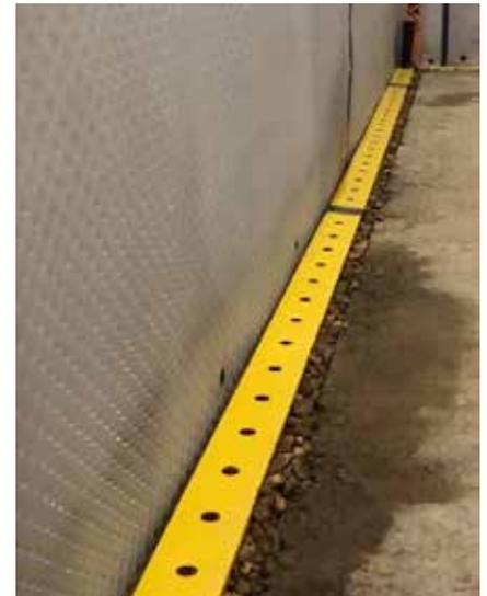
We recommend one Packaged Pump System should be installed for each 50 linear meters of Channel; the length of each Channel running to the Sump should not exceed 25m.
