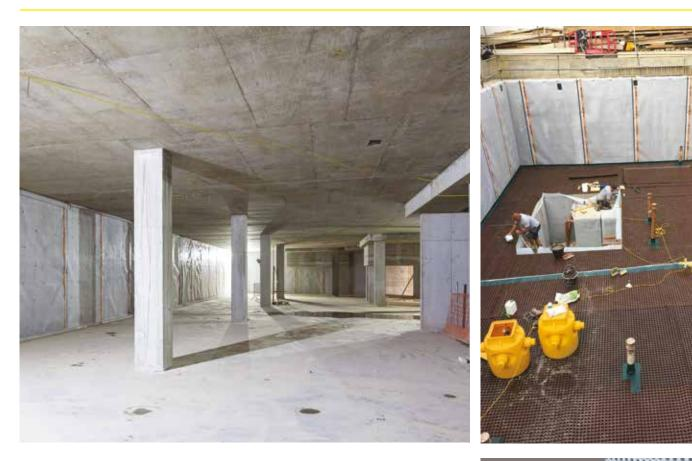
One of the main design considerations when designing a Cavity Drain System is to consider managing the collection and discharge of ground and/or foul water.
