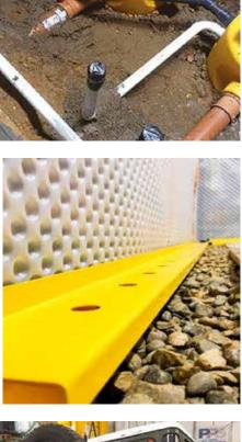
The concept of a Drained Cavity System is to collect and manage any ground water which breaches the integrity of a structure by managing, collecting and discharging such free water via a suitable evacuation point such as a Delta Packaged Pump Station.
