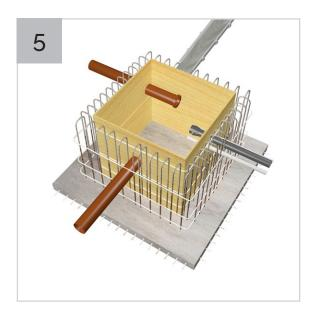
Pour concrete to form the reinforced concrete box as per structural engineer's details.
