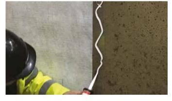
CEM 805 is a one-component, odourless adhesive/sealant that is resistant to weathering and reacts with atmospheric moisture to form an elastic seal. It does not contain solvents, is free of silicone and isocyanates, cures neutrally, is compatible with paints and features excellent chemical resistance.
