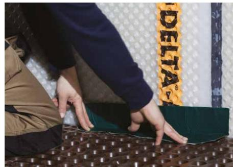
ICF CONSTRUCTION - EXTERNAL WATERPROOFING
