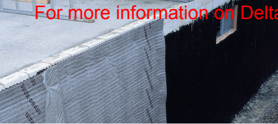
Dependable surface drainage for retaining walls.
