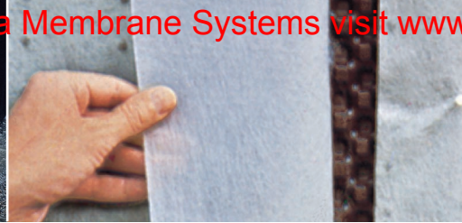
Edge overlap of dimpled sheet and geotextile.
