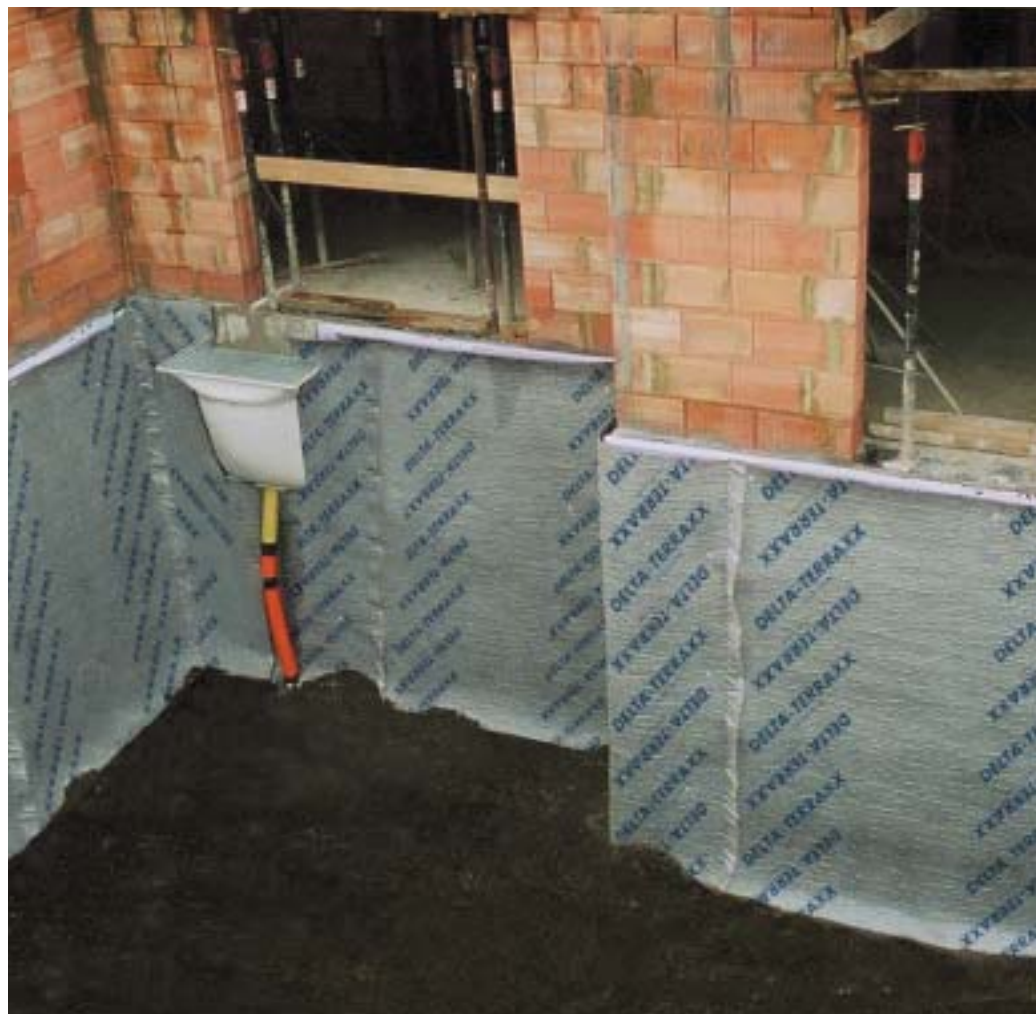
DELTA®-TERRAXX offers permanent-filtration draining.
