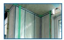
Effisus Adjoin GS Tape is a PE sealing tape with a polyethylene film, as backing.
