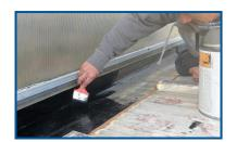
Effisus Coat NP Primer is a ready-to-use sub-coat for absorbent building surfaces. It serves as a bonding agent for the subsequent adhesion of Effisus Ecofacade waterproof facade sealing systems. It promotes adhesion on damp surfaces when using the Effisus Ecofacade Adhesives.
