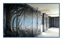
The Effisus Vapour FR is a high quality and multifunctional weatherproofing vapour barrier made of a special fiberglass technology with an aluminum foil, developed to achieve a fire reaction Class A2-s1,d0 according to EN13501-1:2007+A1:2009. The final fire classification was obtained for Effisus Vapour FR with Effisus accessories (tapes and adhesives) tested as a system.
