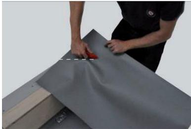
Cut away a section of membrane from the upstand strip.
