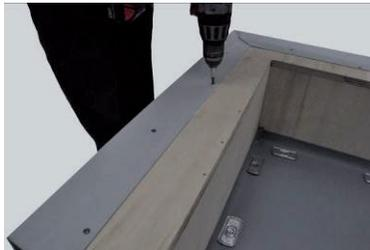
A strip of **RENOLIT** ALKORPLAN D is to be welded over the cut edge.
