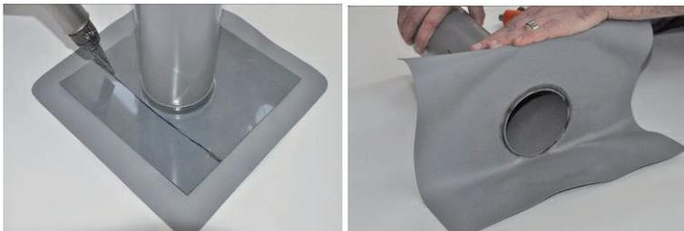
Fasten the prepared outlet (mechanically) to the upstand and weld the flange securely to the field sheet.
