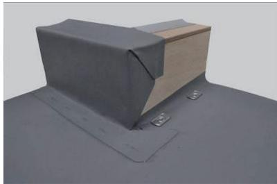
Weld the down the mitre fold to form a pocket. Weld inside the pocket working from the inside outwards
