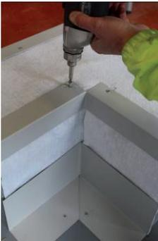
Fix an external ALKORMETAL 50mm x 50mm (minimum) angle to the internal corner.
