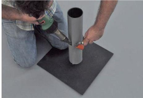
Cut a base flange in **RENOLIT ALKORPLAN D** (unreinforced membrane). The flange must be at least 150 mm larger on all sides of the circumference. Cut a hole in the middle of the flange approximately half the diameter of the pipe.
