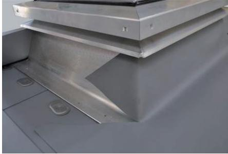
Cut the two remaining upstand strips along the line, as illustrated. Leave a 20 mm 'half round' over to weld the corner and make it waterproof.
