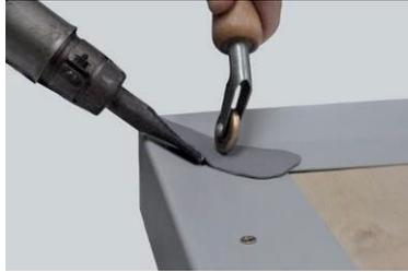
Turn the membranes in the roof deck up by 30 to 50 mm against the upstand and fix along the perimeter edge.
