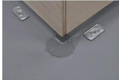
Cut an upstand strip of **RENOLIT ALKORPLAN** of the same height as the upstand to be waterproofed + 100 mm for the overlap with the field sheet.
