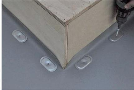
Weld a patch of **RENOLIT ALKORPLAN D** to the apex of the corner.
