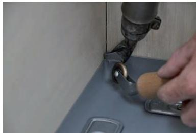
Cut an upstand strip of **RENOLIT ALKORPLAN** the same height as the upstand to be waterproofed + 100 mm for overlap with the field sheet.
