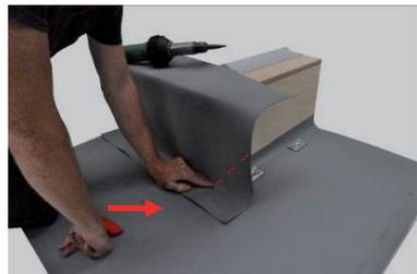
Detach the locating welds on the **RENOLIT** ALKORPLAN metal sheet profile and apply contact adhesive to the entire face of both the upstand and upstand strip. Free any creases around the corner. Allow time for the adhesive to go tacky on both faces then smooth the membrane into place and weld the upstand strip fully and securely to the metal edge profile.
