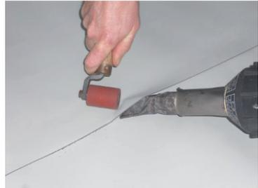
**Apart from initially maintaining material in position, Spot welds are unacceptable.**
