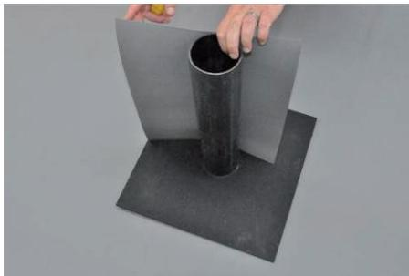
This strip is glued around the pipe using **RENOLIT ALKORPLUS** 81040 contact adhesive. The overlap is hot-air welded on the vertical lap.
