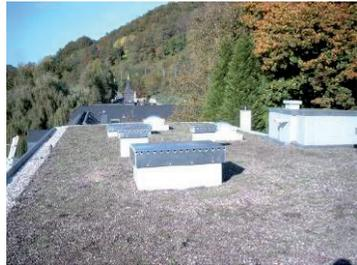
The ballast layer should be applied immediately after the **RENOLIT ALKORPLAN L** roofing membrane and its protection layer in order to offset wind forces.
