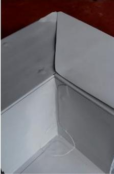
Weld **RENOLIT** ALKORPLAN membrane to the horizontal faces of the ALKORMETAL drip and angle.
