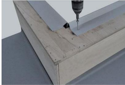
Cover the exposed part of the corner by welding a patch of **RENOLIT ALKORPLAN D** on top.
