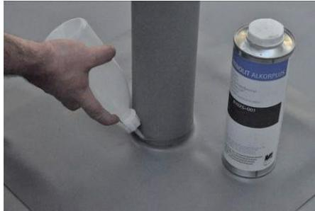
Weld the **RENOLIT** ALKORPLAN D flange to the field sheet with a minimum width of 40 mm around the perimeter.
