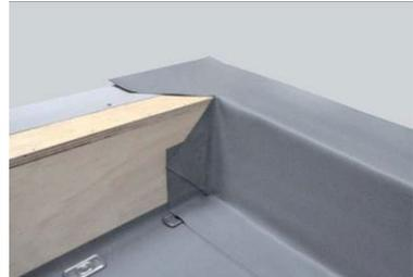
Follow the same procedure for the adjacent upstand. Cut the sheet into the corner as shown.
