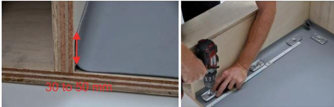
**Please note: As an alternative method of perimeter fixing a peel stop bar may be installed along the edge, RENOLIT ALKORPLUS<sub>81103</sub>.**
