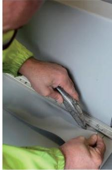
The fold in the corner should be welded using a manual hot air gun.
