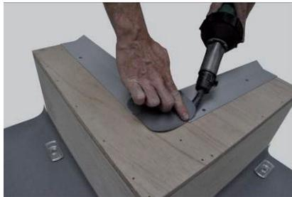
Turn the membranes in the roof deck up by 30 to 50 mm against the upstand and install an edge restraint.
