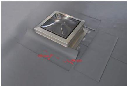
Apply **RENOLIT ALKORPLUS<sub>81040</sub>** contact adhesive to two opposing sides of the skylight dome and to two cover strips.
