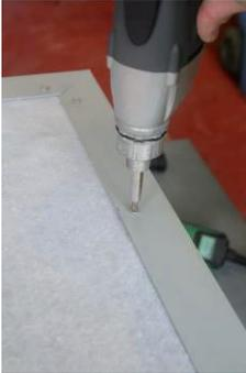
Cut the ALKORMETAL drip section so it fits onto an external corner and fix it to the substrate.
