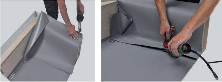
Weld the upstand strip onto the field sheet, to form an upright fold in the corner.
