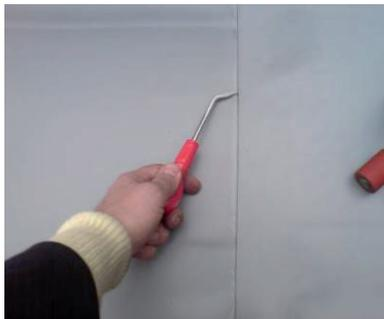
Any un-welded overlaps must be re-welded immediately with hot air.
