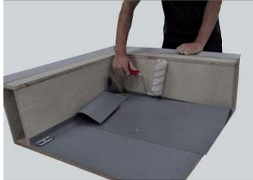
Weld up the fold to form a waterproof pocket. Work from the inside outwards.
