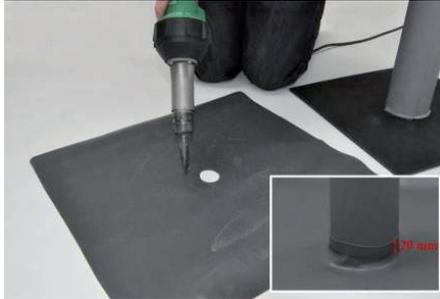
Weld the 20 mm lip using **RENOLIT ALKORPLUS<sub>81025</sub>** solvent and finish the seam with seam sealer.
