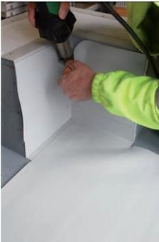
Weld the field sheet to the base of the ALKORMETAL leaving a gap of 20mm between the edge of the membrane and the vertical face of the profile.
