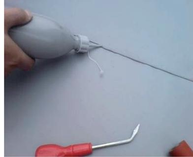
Ensure that the membrane is clean and dry before using seam sealer.
