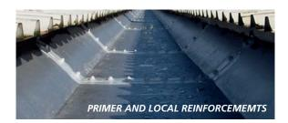
The Elastex 15 Year System was installed to provide a fully seamless waterproofing solution. Daily operations at the company were unaffected by the works, adding further value to the decision to overlay the gutter.
