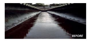
The rust in the gutters was ground out and then treated with a rust converter. The gutter was primed with metallic primer and local reinforcements to the bolt heads and lap joints were carried out.
