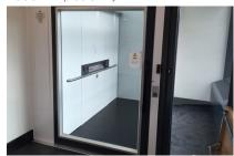
A heavy duty platform lift suitable for passengers, wheelchair users, bikes and goods. Travels up to 13m with 1000kg lifting capacity & larger clear door opening sizes into the platform lift for goods movement.
