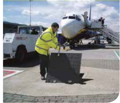
Two-part solid-top cover - Type SSA These are fitted with a removable central support bar.
