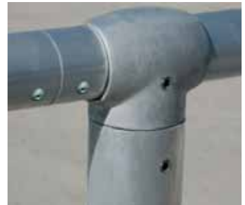
mechanical fixings to all connections
