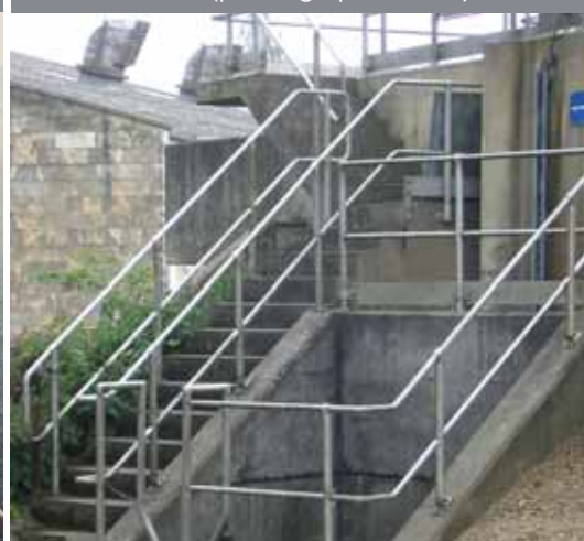
Tadcaster Water Treatment Works
