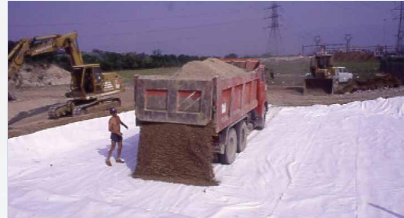
Its soft, cushioning properties mean it can be placed onto rough areas to prevent sharp objects from passing through into the system above but still allow the passage of water. This means sealing and waterproofing sheet membranes can be installed above them without the risk of ground settlement causing any damage above.
