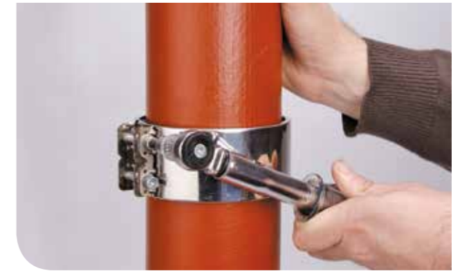
4. Evenly tighten the bolts to the required torque setting. The coupling should only be tightened once, because it cannot be dismantled and re-used. (See Couplings Data page 55)
