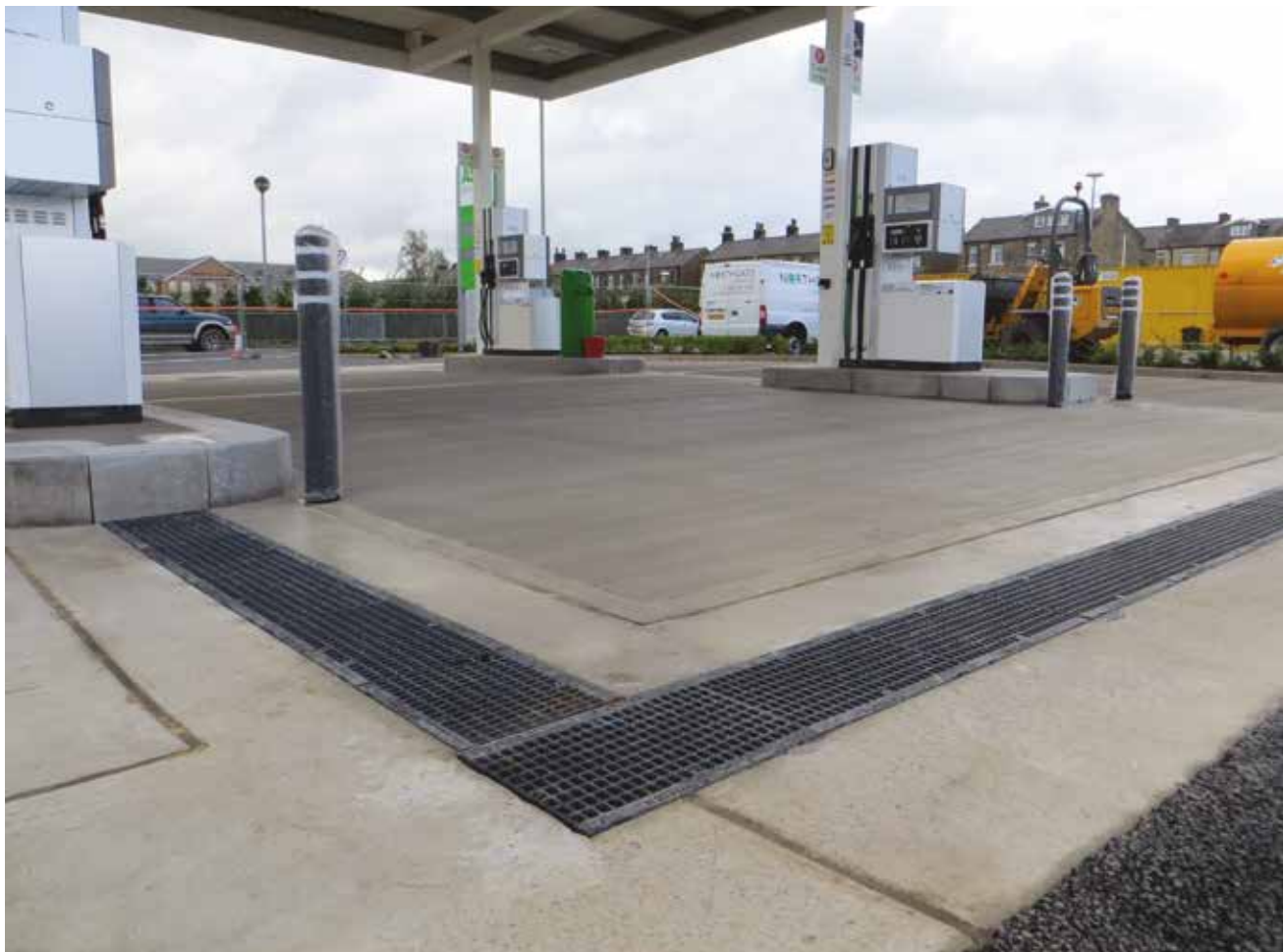
Petrol Filling Station , Dewsbury, Yorkshire
