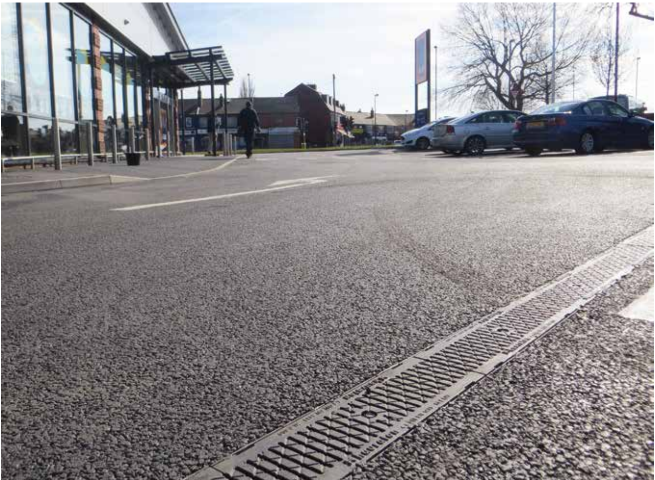
Car Park Middleton Leeds
