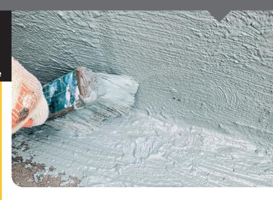
HydraFlex is a two-component flexible coating made of a cementitious powder and a high concentration liquid polymer.
