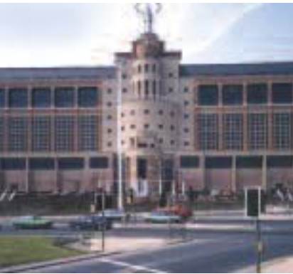
The DHSS Building, Leeds. Just one of the many prestigious projects where the designers called on the DPC expertise of Icopal. For more information see pg 11.
