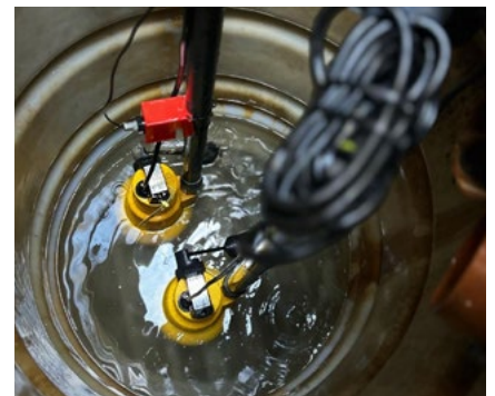
Sump pumps in chamber after service
