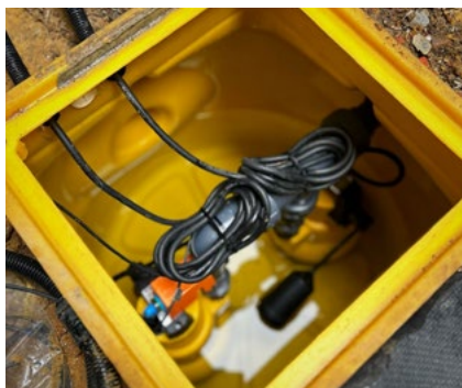
Dual V3 pumps in chamber after service
