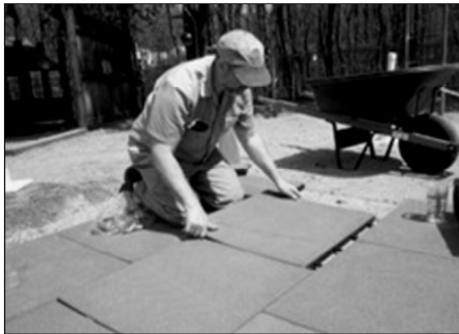
Playground Tile Installation
