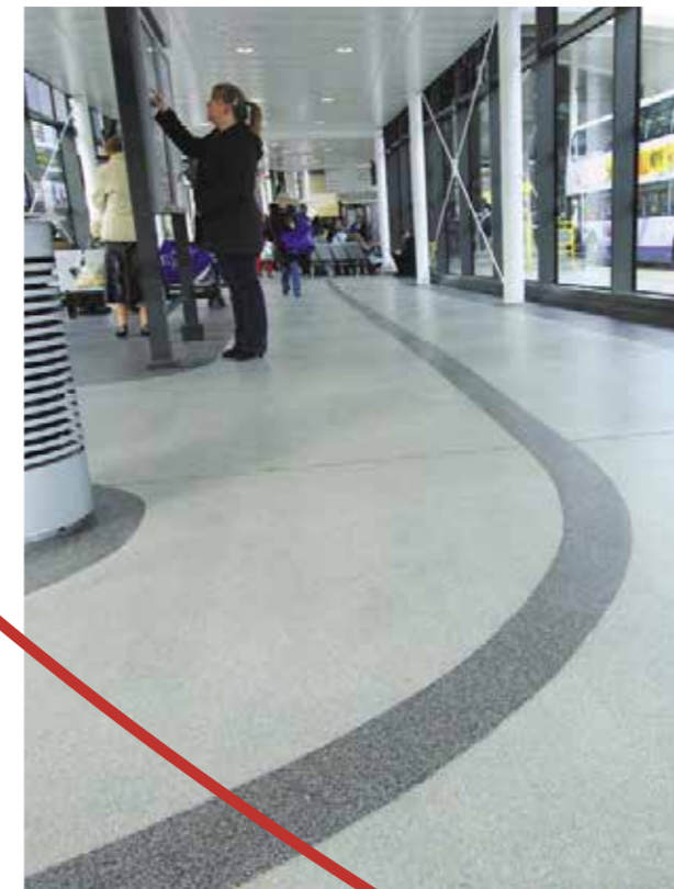
Rochdale Bus Station using Acrigard QB
