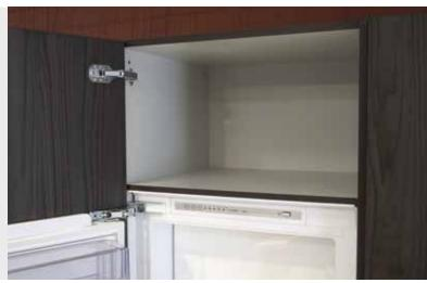
However, these extra high fronts create the problem of the top part of the door not having any stability when it is opened. The springless Kamat guiding hinge was developed to permit stable reveal alignment.
