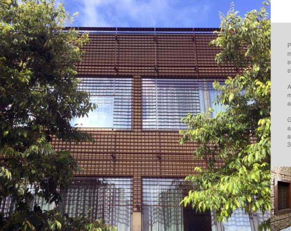
Panels of Corten grating are manufactured to custom-sizes and supplied framed with supporting steel work and fixings as required.
