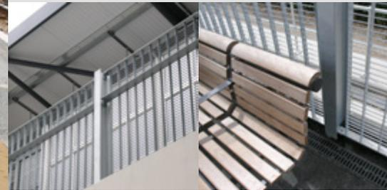
**Case Study:** Torino-33 was designed to meet Network Rail's requirements for a barrier fence at a new station at Rochester. The brief was to supply fencing which would sustain a crowd loading while providing an uninterrupted view of the town's historic buildings.
