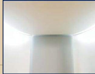
controllable dimmed ceiling downlighting
