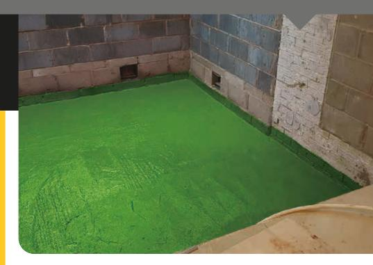
Wykamol Liquid Gas Membrane (LGM) is a single pack, elastomeric liquid rubber membrane, specifically designed for a range of vertical and horizontal construction surfaces, generally as follows. LGM will cure to form a tough, flexible material acting as an effective barrier to the passage of vapour, damp, water, Radon and Methane gas.
