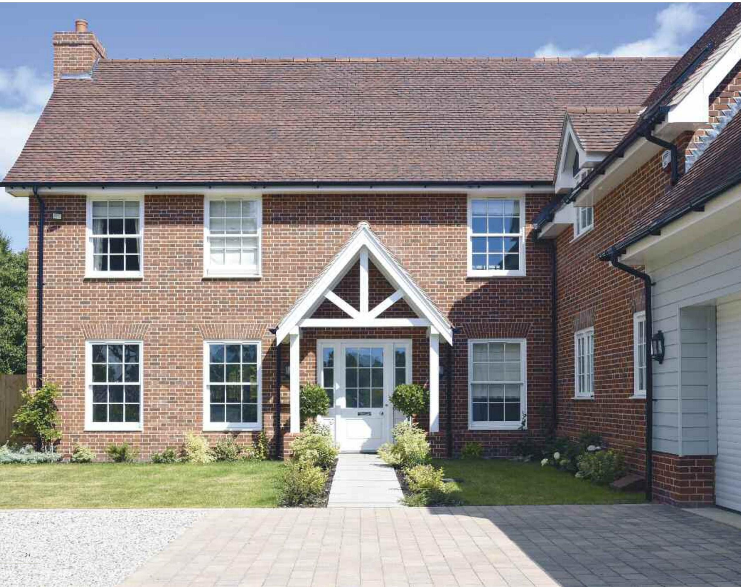
These specially adapted sash windows are hung on pre-tensioned springs and have a tilt and slide bottom sash which efficiently and conveniently tilts inwards into the room. Externally the window coordinates with all products in the Conservation™ collection, has slender meeting rails, fine glazing bars and traditional mouldings.
