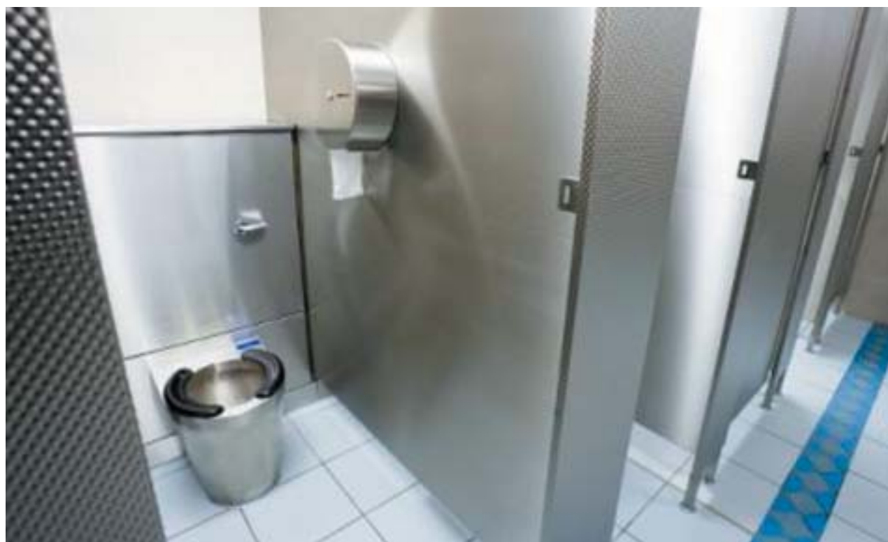
Olympic anti-vandal stainless steel WC pan. Stainless steel clad cubicles.
