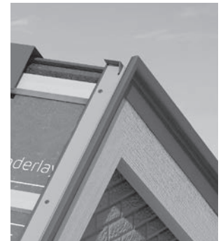
Fig. 27 – Interlock left and right hand trims
