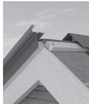
Fig. 26 – Nail left hand trim in place
