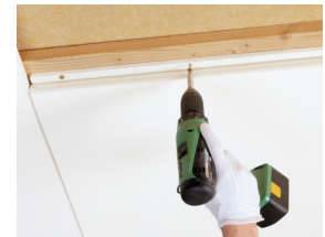
Master F is installed by screw fixing
