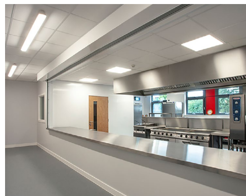
Fig. 2 Suspended fitting with 30:70 uplight / downlight. The light on the ceiling reduces the contrast, so the glare is reduced.
