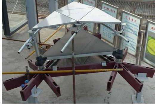
Fig. 5: Freeform Roof Built-Up Mockup
