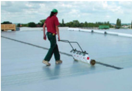
Pict. 1: Application of the polyurethane glue by means of an applicator
