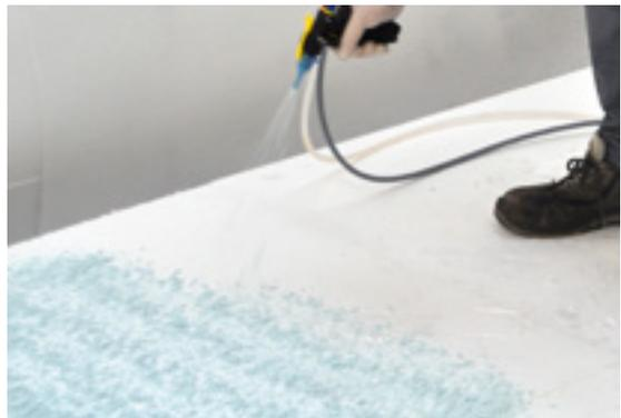
Pict. 2: The adhesive RENOLIT DUALFIX<sub>81065</sub> is atomized by means of a spray gun.
