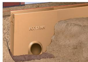
Lay channels starting from outlet/sump, ensuring joints connect by lowering units horizontally. Fit endcap to end channel. For fully watertight joints, use a suitable sealant (contact ACO for further advice).
