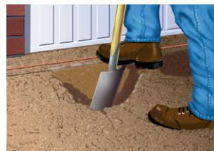
Dig trench 318mm wide (218mm wide if against a structure) by 200mm deep for channel (400mm deep for sump). Mark finishing height with fixed line 3mm below final surface. Lay 100mm (min.) bed of concrete.
