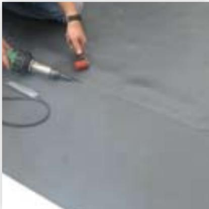
The **SPEED** at which the welding gun is moved
