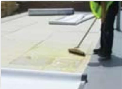
When the adhesive is applied in lines, as illustrated, it must be squeegeed across the width of the membrane to create a full bond.
