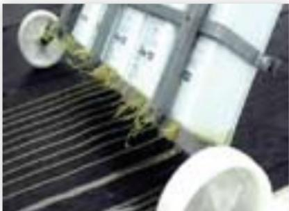
The amount of glue to be used is specified by the wind load calculation carried out by a qualified engineer.
