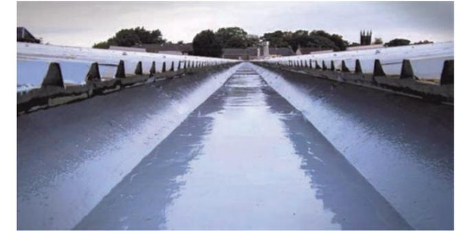
The tough elastomeric membrane provides a resilient long lasting barrier to water and its flexibility easily accommodates normal expansion movements. Elastex can be applied direct to the metal substrate for a rapid refurbishment with minimum disruption.
