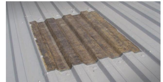
Transglaze has been specially formulated to permit the continuous transmission of light into the building. When used in conjunction with Roofcoat Plus, the systems form a totally seamless waterproof membrane that provides a long-lasting barrier to water.
