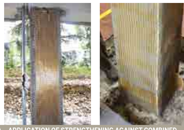
APPLICATION OF STRENGTHENING AGAINST COMBINED AXIAL AND BENDING FORCES, SHEAR, AND CONFINEMENT
