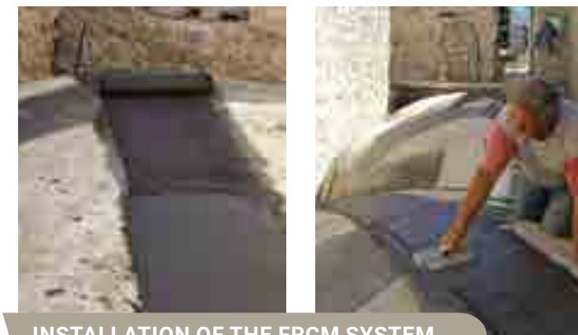
INSTALLATION OF THE FRCM SYSTEM
