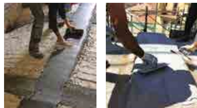
INSTALLATION OF THE FRCM STRENGTHENING
