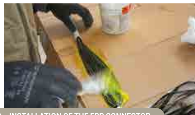
INSTALLATION OF THE FRP CONNECTOR
