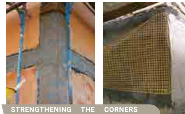
STRENGTHENING THE CORNERS AND FLOOR EDGE BEAMS
