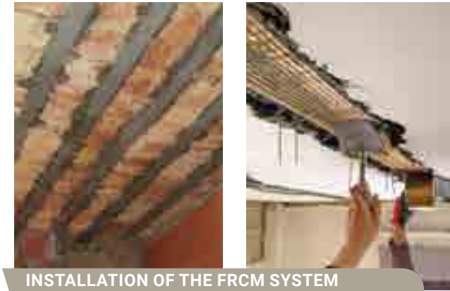
INSTALLATION OF THE FRCM SYSTEM TO THE INTRADOS OF THE JOISTS
