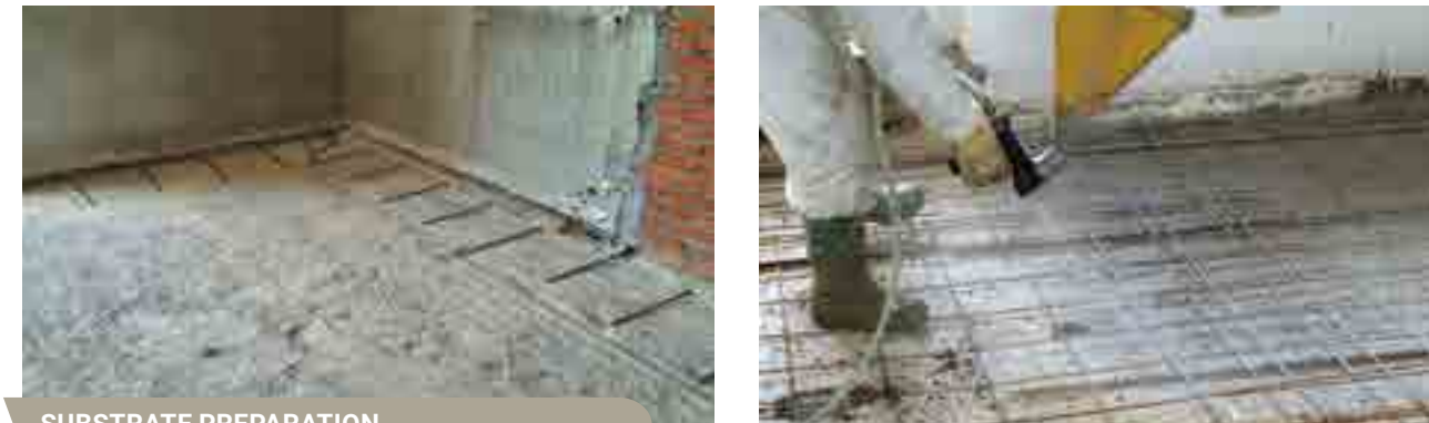
SUBSTRATE PREPARATION
