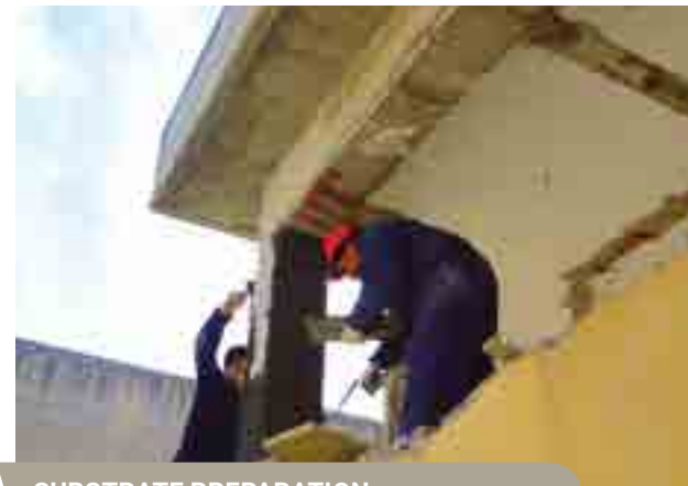
SUBSTRATE PREPARATION
