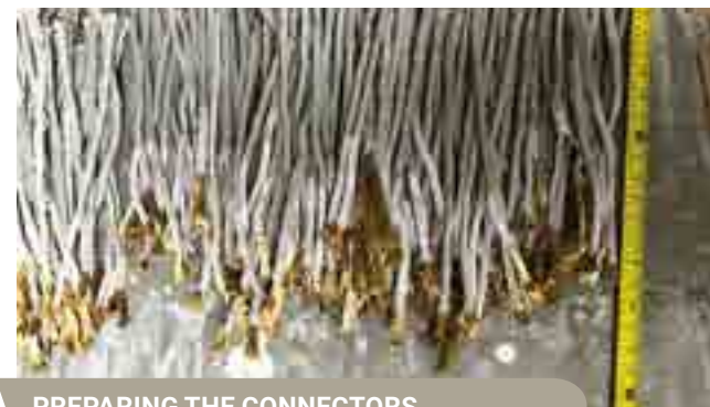
PREPARING THE CONNECTORS
