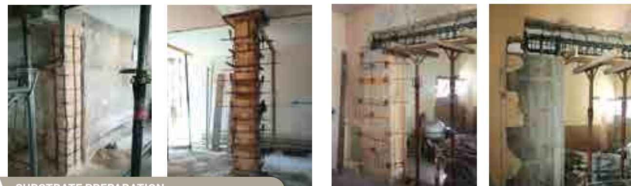
SUBSTRATE PREPARATION
