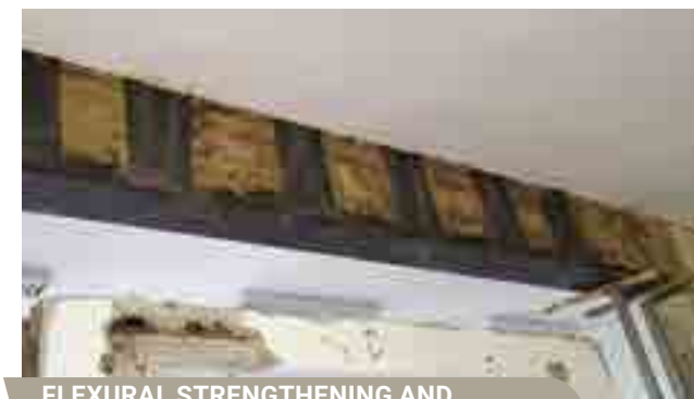
FLEXURAL STRENGTHENING AND SHEAR STRENGTHENING WITH STRIPS
