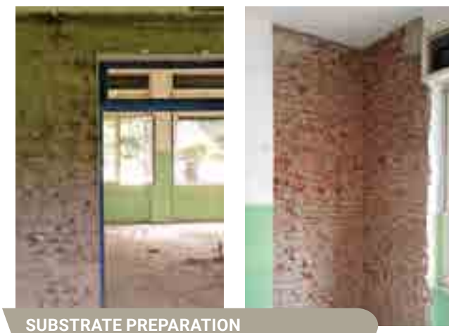
SUBSTRATE PREPARATION
