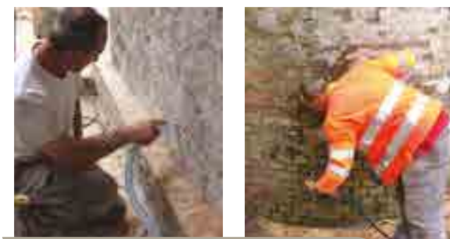
INJECTION OF BINDING MIXTURES
