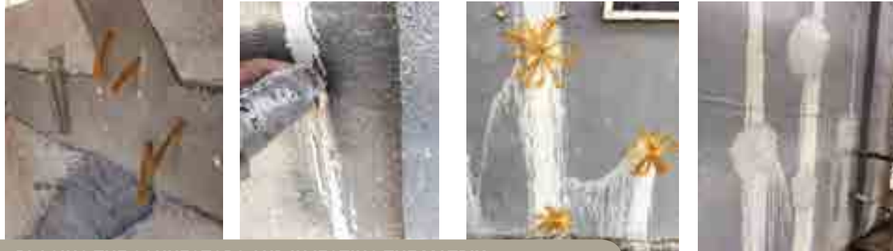
PLACING THE CONNECTORS AND INJECTING THE MATRIX
