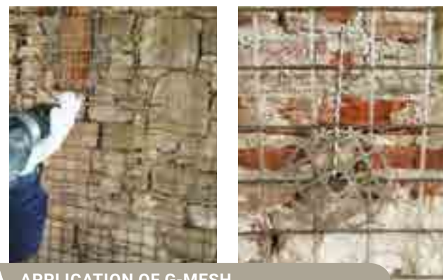
APPLICATION OF G-MESH
