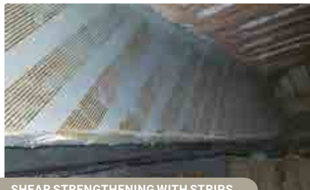
SHEAR STRENGTHENING WITH STRIPS
