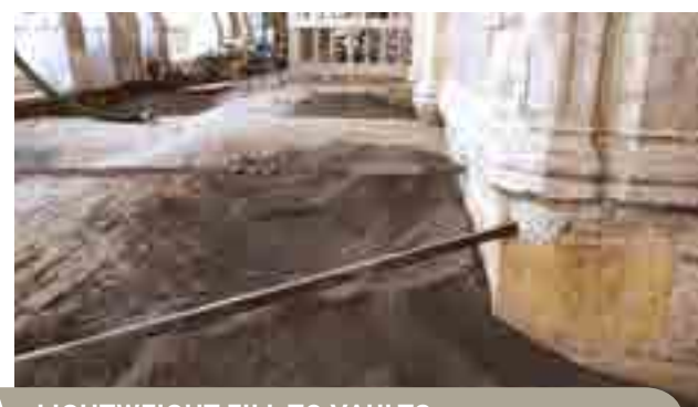
LIGHTWEIGHT FILL TO VAULTS
