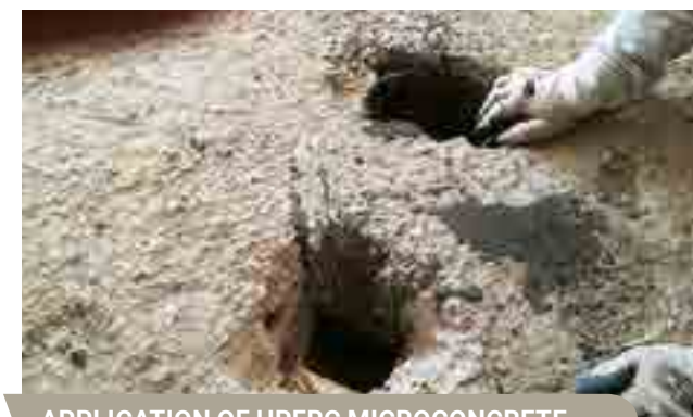
APPLICATION OF HPFRC MICROCONCRETE
