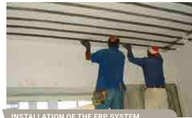
INSTALLATION OF THE FRP SYSTEM
