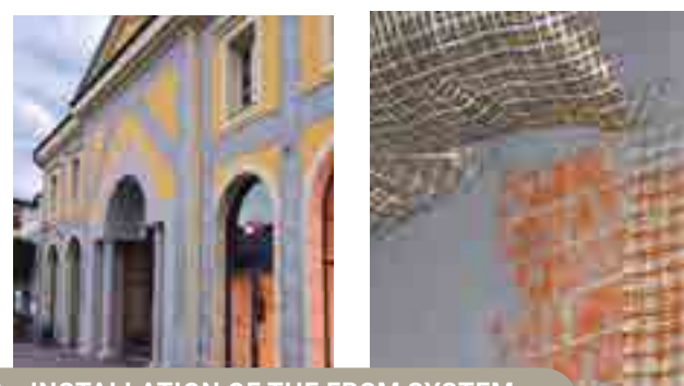
INSTALLATION OF THE FRCM SYSTEM
