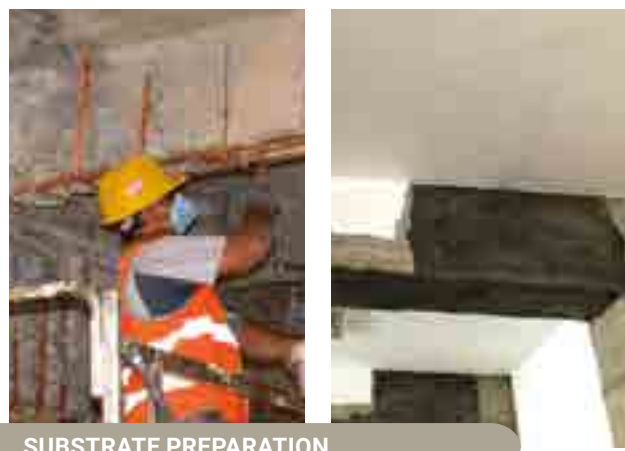
SUBSTRATE PREPARATION
