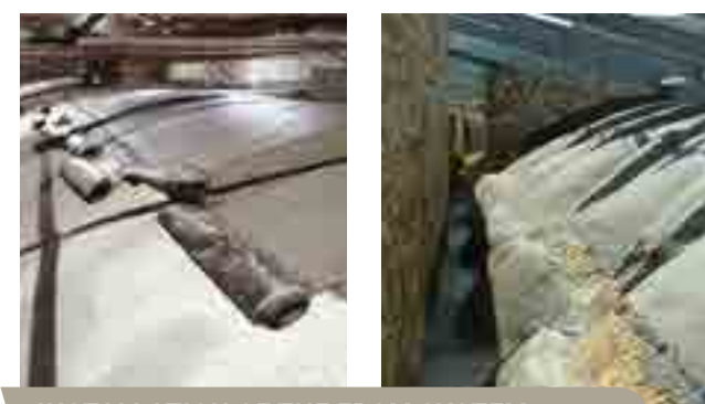
INSTALLATION OF THE FRCM SYSTEM
