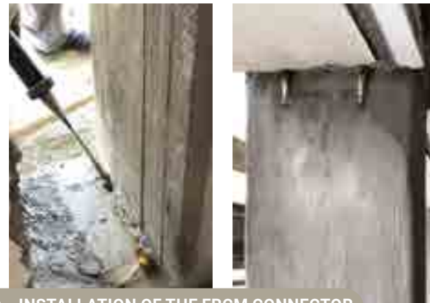
INSTALLATION OF THE FRCM CONNECTOR
