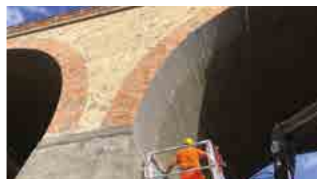
INSTALLATION OF THE FRCM STRENGTHENING
