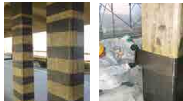
FRP SHEAR AND CONFINEMENT STRENGTHENING
