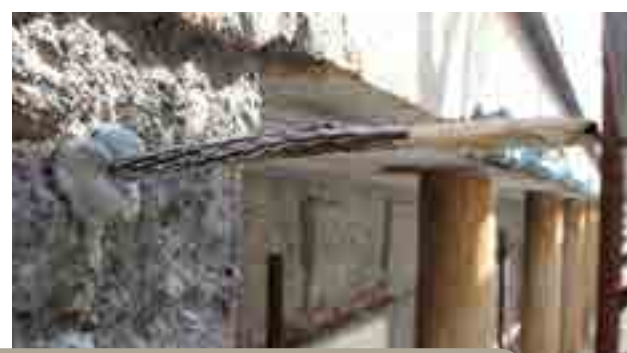
INSTALLATION OF THE CONNECTOR
