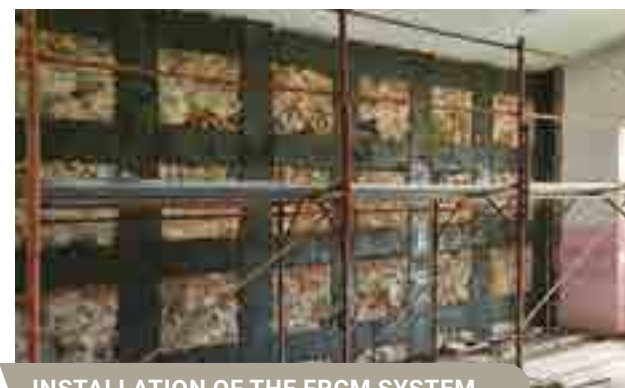
INSTALLATION OF THE FRCM SYSTEM
