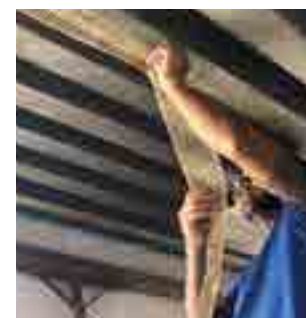
INSTALLATION OF THE FRCM SYSTEM
