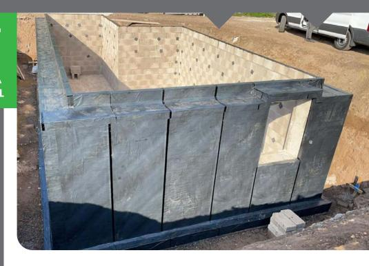
The high-density polyethylene film gives to the membrane characteristics of dimensional stability and ensures a uniform reaction to elongation stresses in a longitudinal and transversal direction.
