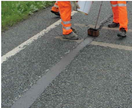
SAFETRACK® INLAID ROAD REPAIR APPLICATION
