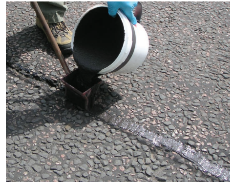
SAFETRACK® OVERBANDING APPLICATION
