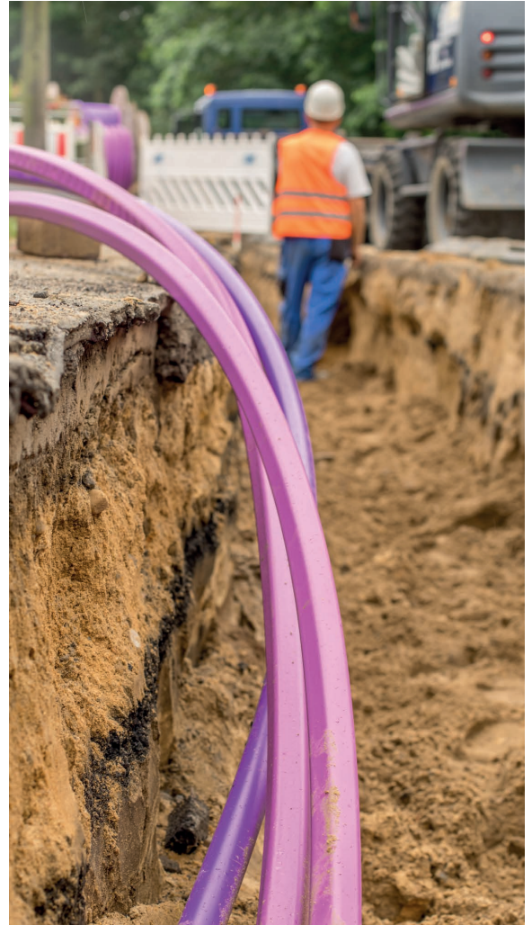
HIGHWAY REINSTATEMENT WORKS
