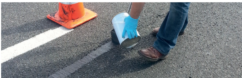
SAFETRACK® CRACK INFILL APPLICATION
